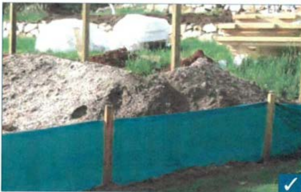
Figure 7: Correctly installed sediment fence
