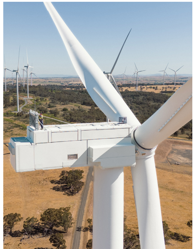
Bango Wind Farm near Boorowa NSW
