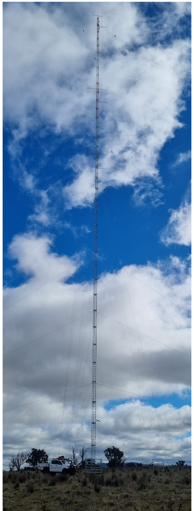
A wind monitoring mast
