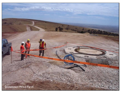
Typical hardstand area adjacent to a rock anchor footing
