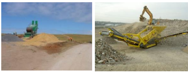
Temporary on-site concrete batching plant and rock crusher
