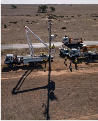
Installation of overhead transmission lines
