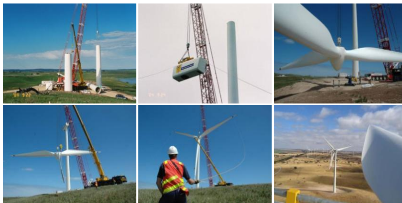
A range of typical turbine erection photographs
