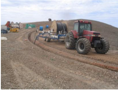
Laying underground electrical cable within road network
