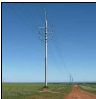
Image 3.6 Double-circuit overhead 33 kV transmission line
