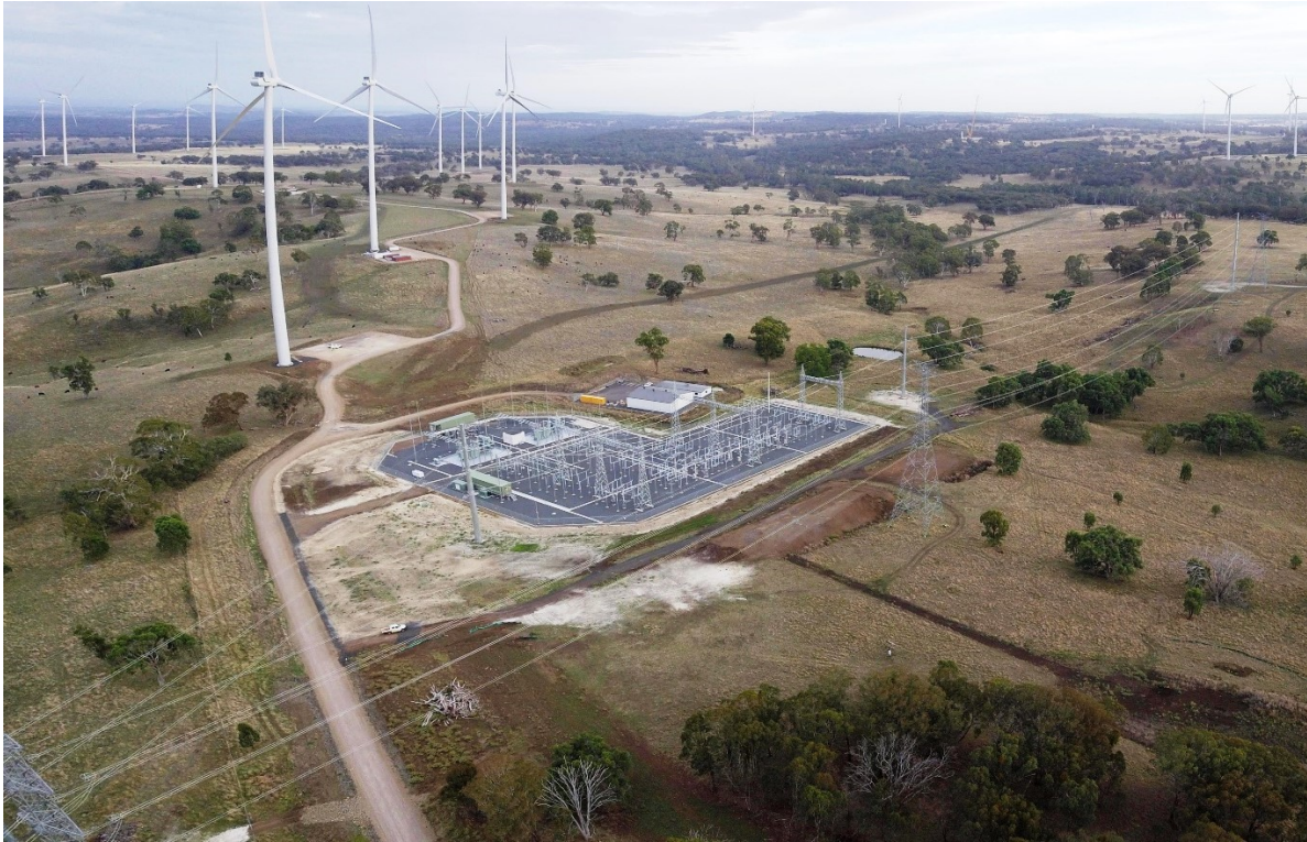
Figure 2.6: Example of a 270 MW Wind Farm Substation
