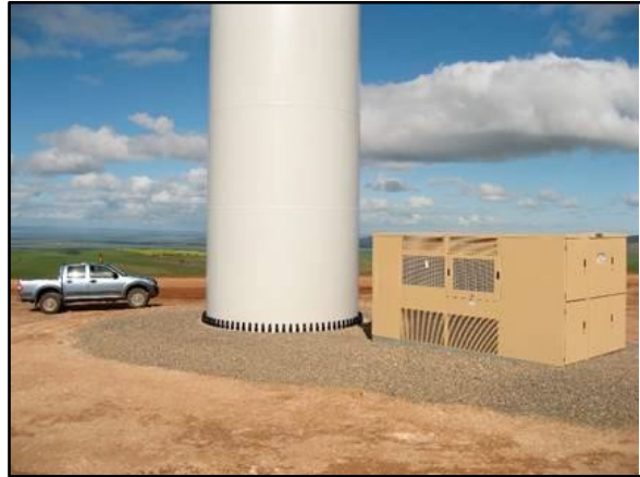
Figure 2.10: Gravel dressing around wind turbine base, with external transformer kiosk 4
