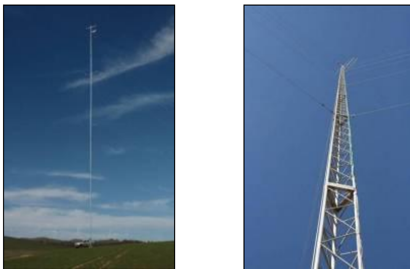
Image 3.4 Tubular (left) and lattice (right) wind monitoring masts
