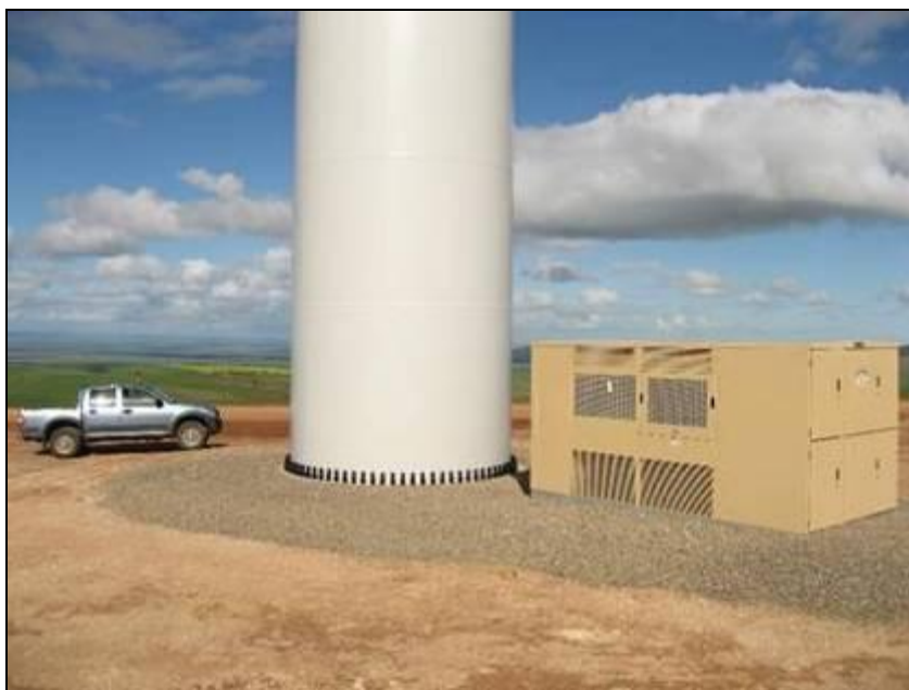
Image 3.5 Transformer adjacent to wind turbine
