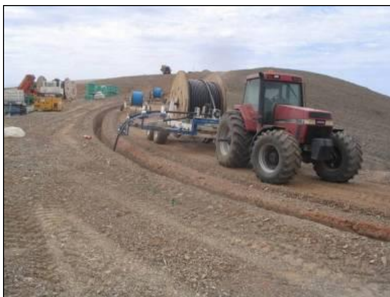
Image 3.7 Laying underground transmission line within the road network
