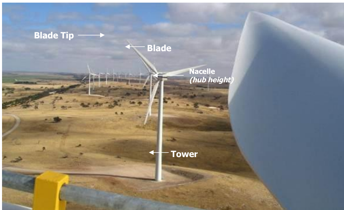
Image 3.1 Components of a wind turbine
