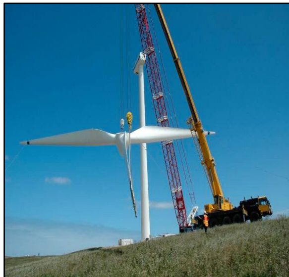
Figure 2.11: A typical wind turbine rotor installation 5
