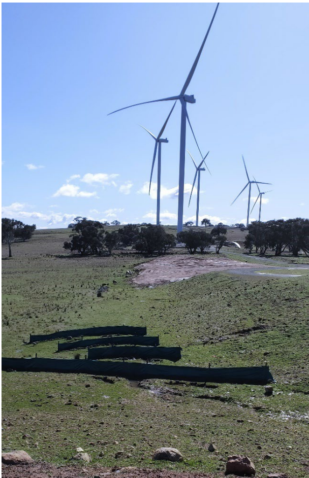
Photograph C.2 Sediment control, grass area re-established
