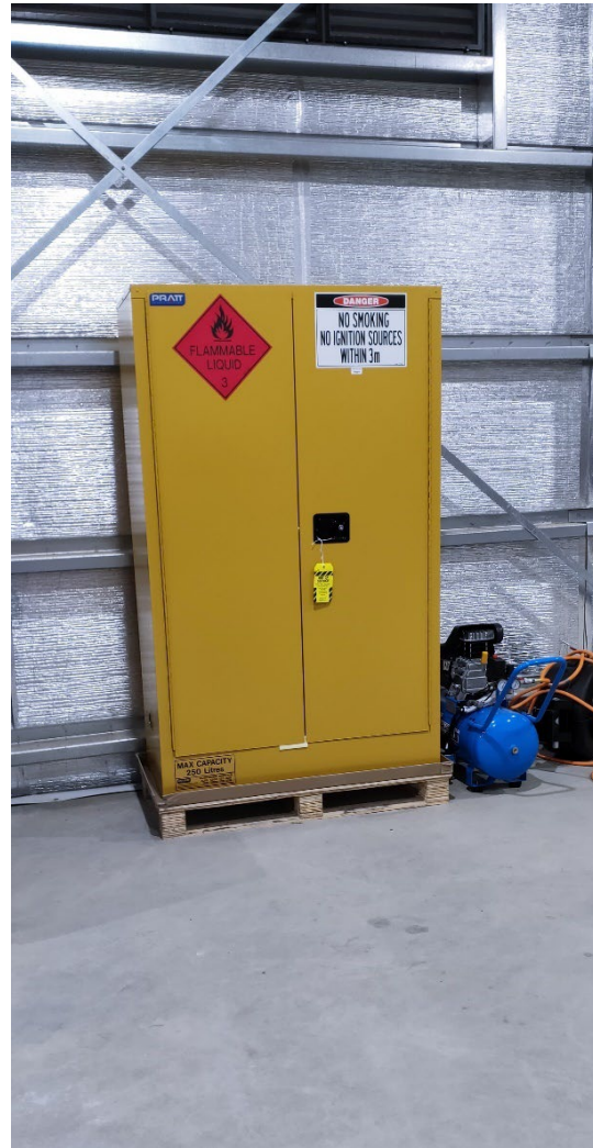
Photograph C.10 Lockable, self-bunded flammable goods storage well managed on site
