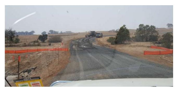
Photograph D.7 Water Cart in use near active construction area
