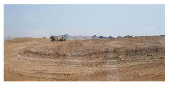
Photograph D.8 Stockpile area setup of erosion controls (bunded areas installed as slope breaks)
