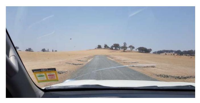
Photograph D.13 Completed access road area with erosion controls and final road surface. Approved 200m corridor flagging visible on the left and right edges
