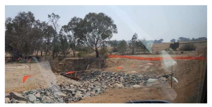
Photograph D.6 Creek crossing under construction. Scour protection installed and pipe crossing in place
