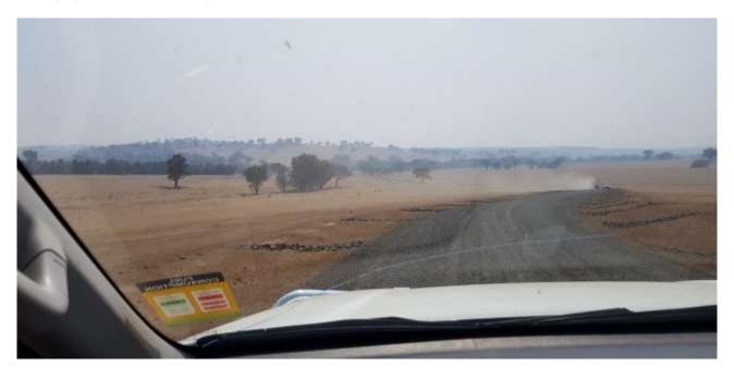
Photograph D.2 Dust from vehicle on final road surface. Limited water used on final surface due to very low water supply
