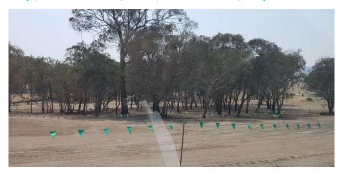
Photograph D.10 Retained vegetation delineated with flagging
