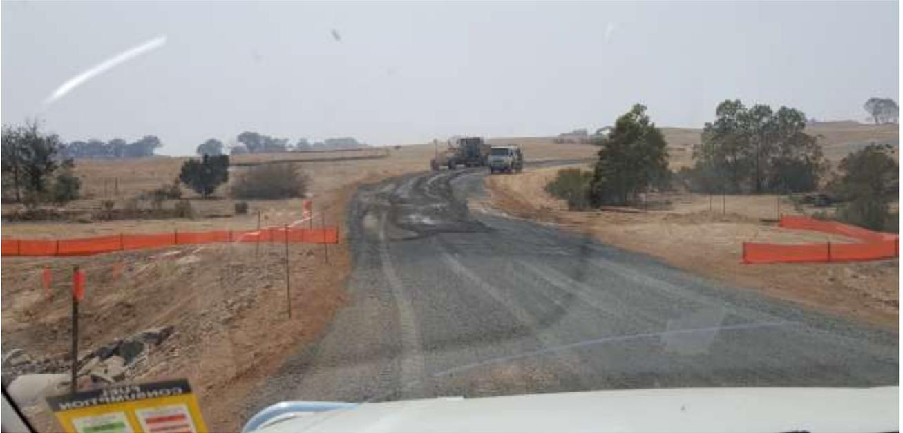
**Photograph D.7** Water Cart in use near active construction area
