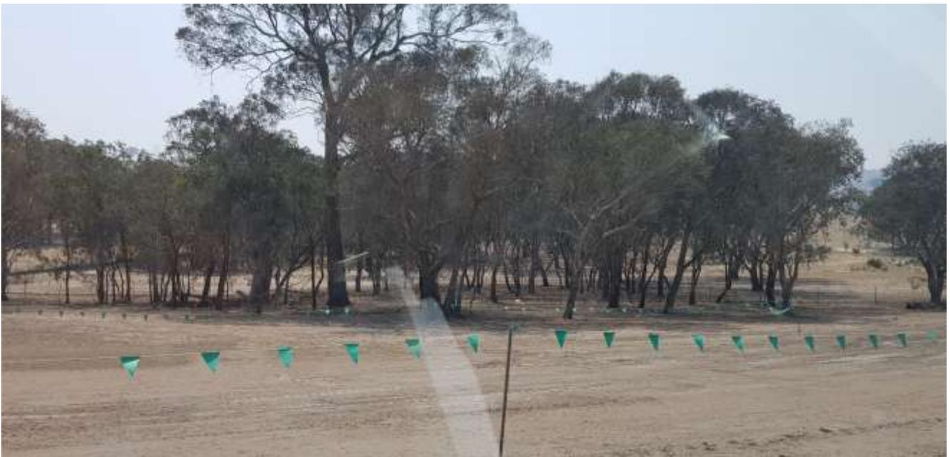
**Photograph D.10** Retained vegetation delineated with flagging
