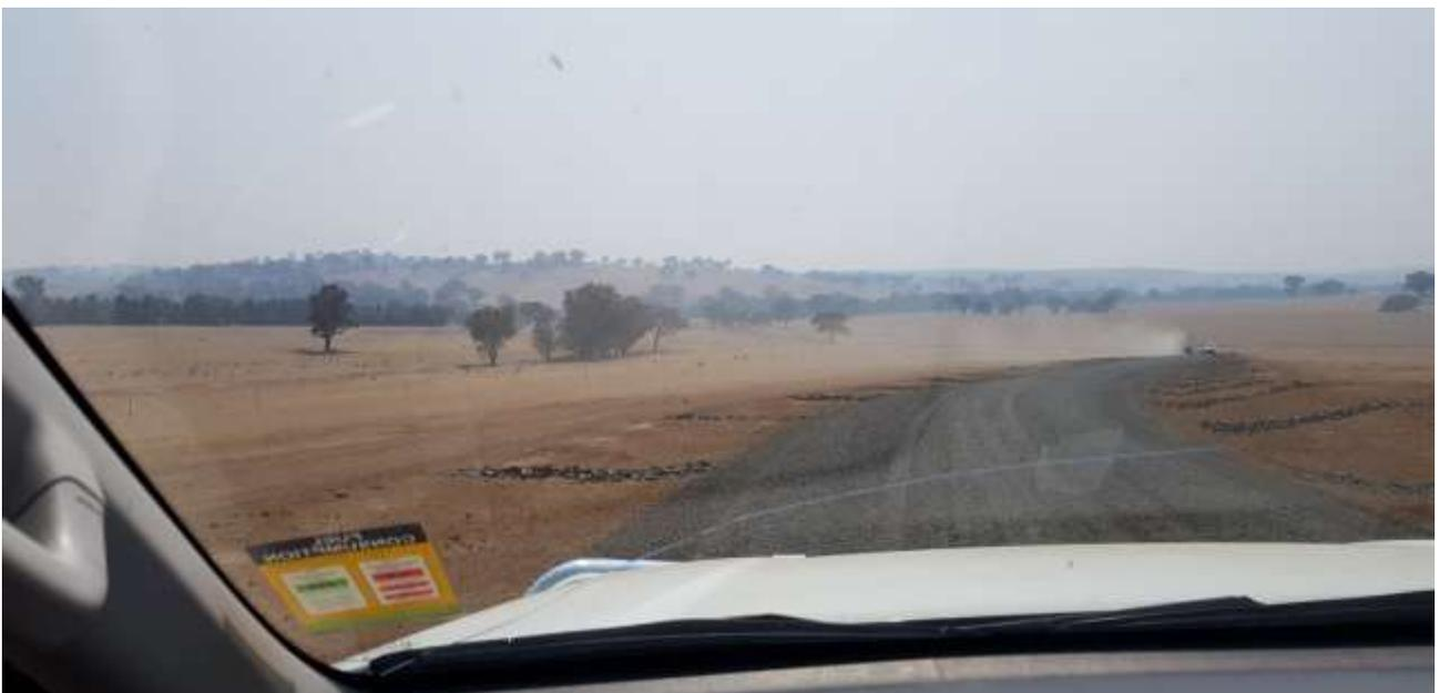
**Photograph D.2**      **Dust from vehicle on final road surface. Limited water used on final surface due to very low water supply**
