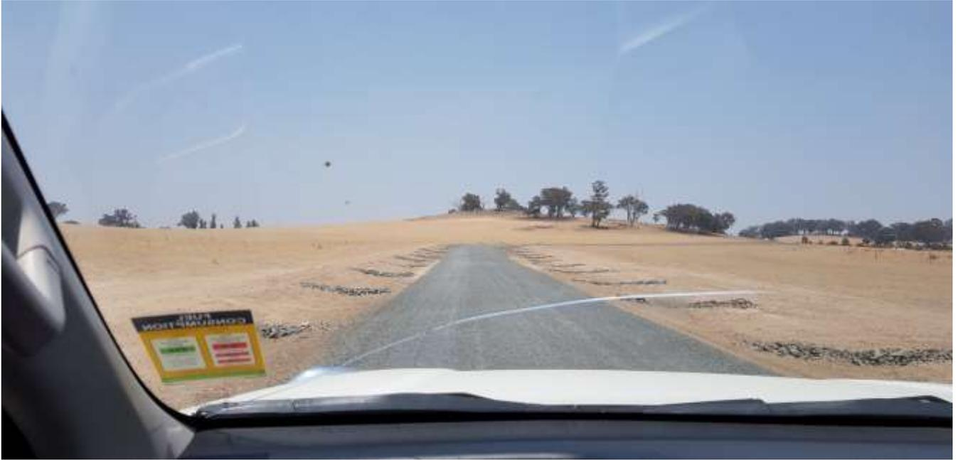
**Photograph D.13** Completed access road area with erosion controls and final road surface. Approved 200m corridor flagging visible on the left and right edges
