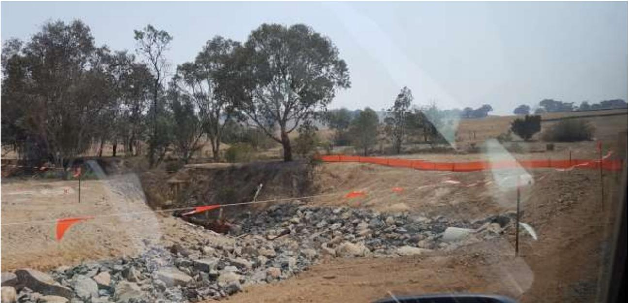
**Photograph D.6** Creek crossing under construction. Scour protection installed and pipe crossing in place
