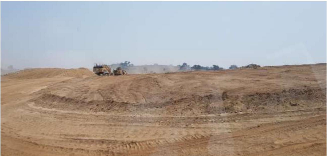
**Photograph D.8** Stockpile area setup of erosion controls (bunded areas installed as slope breaks)
