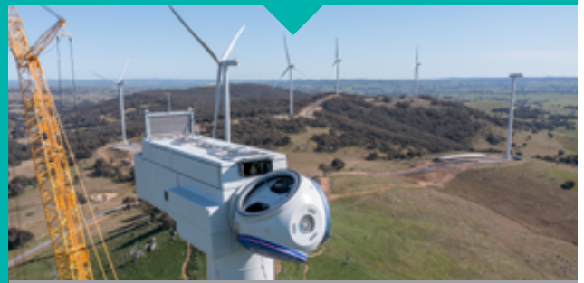
Construction in the eastern cluster continues.
