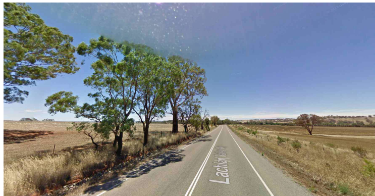
SIGHT DISTANCE NORTH
