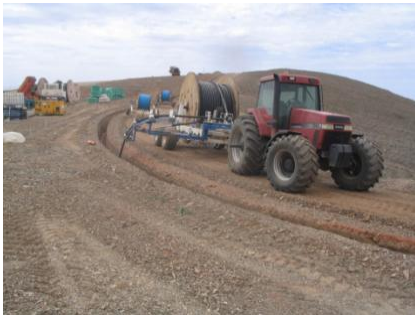
Laying underground electrical cable within road network
