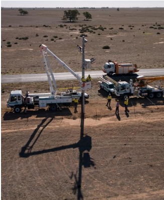
Installation of overhead transmission lines
