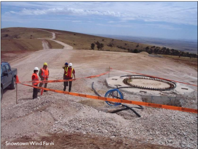
Typical hardstand area adjacent to a rock anchor footing
