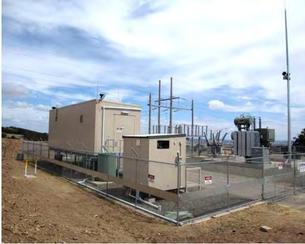
Plate 7 – Typical wind farm collector substation
