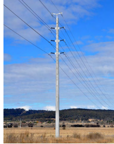
Plate 8 – Typical illustration of a 132 kV double circuit powerline
