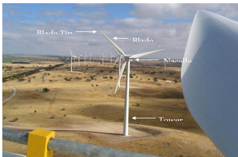
Photograph 2.1 Components of a Wind Turbine
