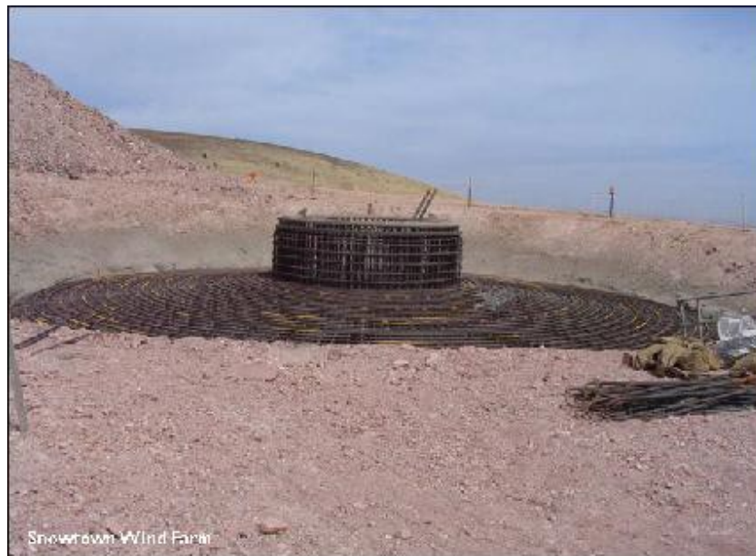
Photograph 2.2 Typical Gravity Footings
