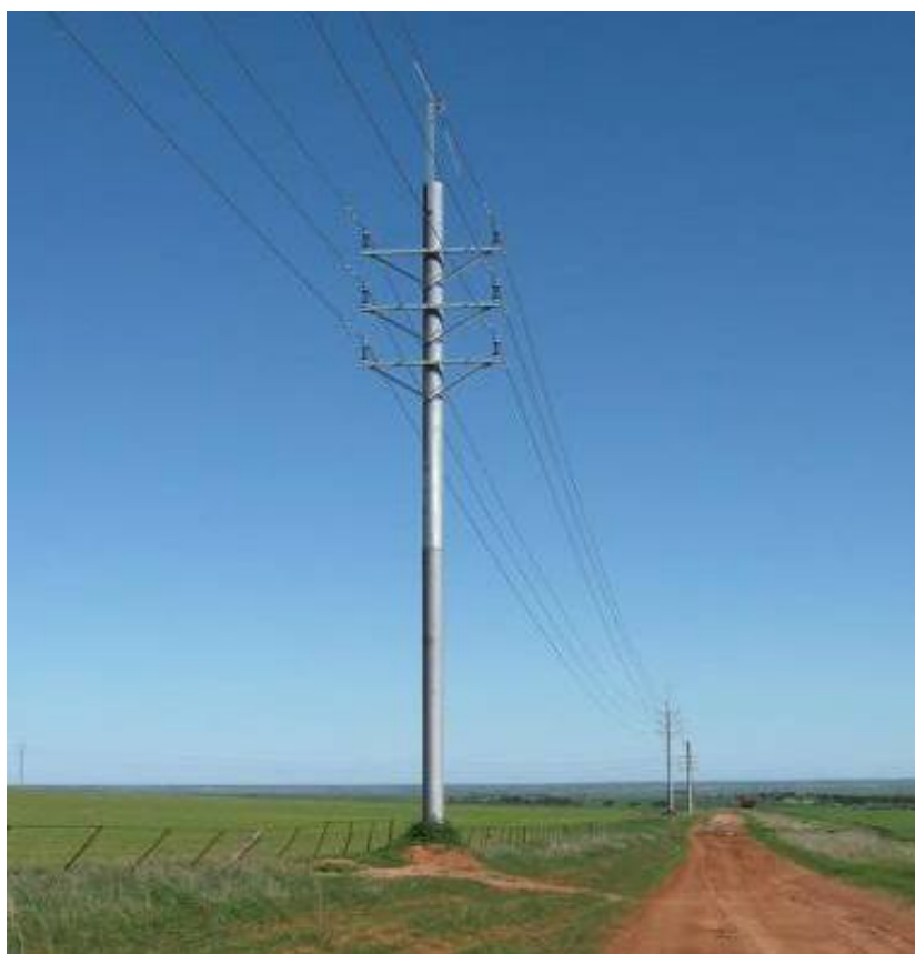
Photograph 2.4 Double-circuit overhead 33 kV transmission line
