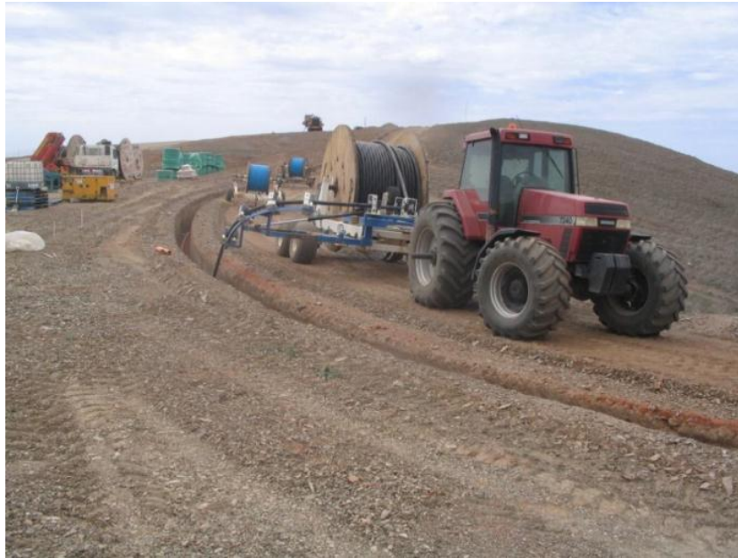
Photograph 2.5 Laying underground transmission line within the road network
