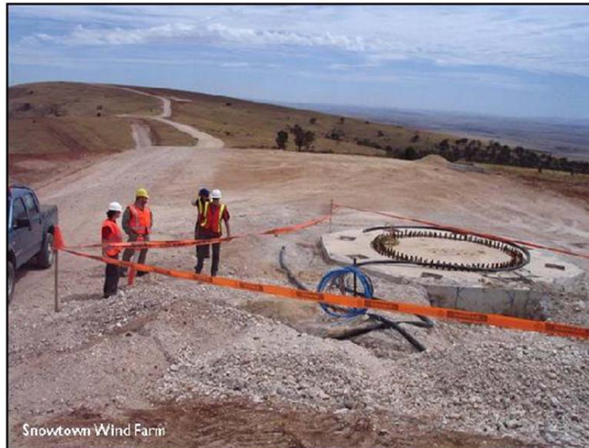
Photograph 2.3 Typical hardstand area adjacent to a rock anchor footing
