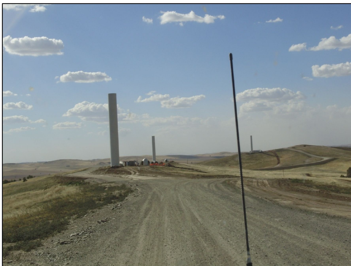
Figure 5.1: Typical unsealed access road within wind farm site
