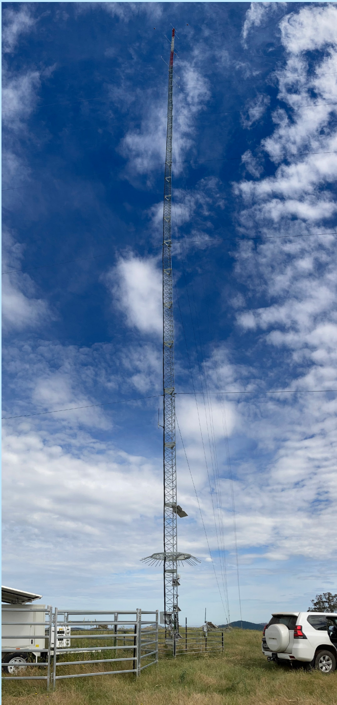
A meteorological mast is used to monitor wind speeds and directions
