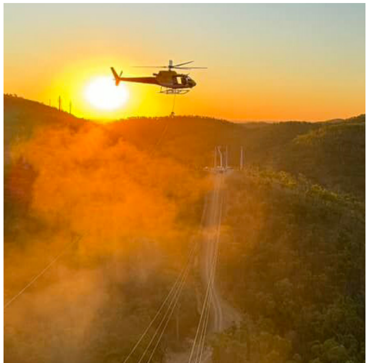
Heli-stringing operation performed by the specialist helicopter and crew.
