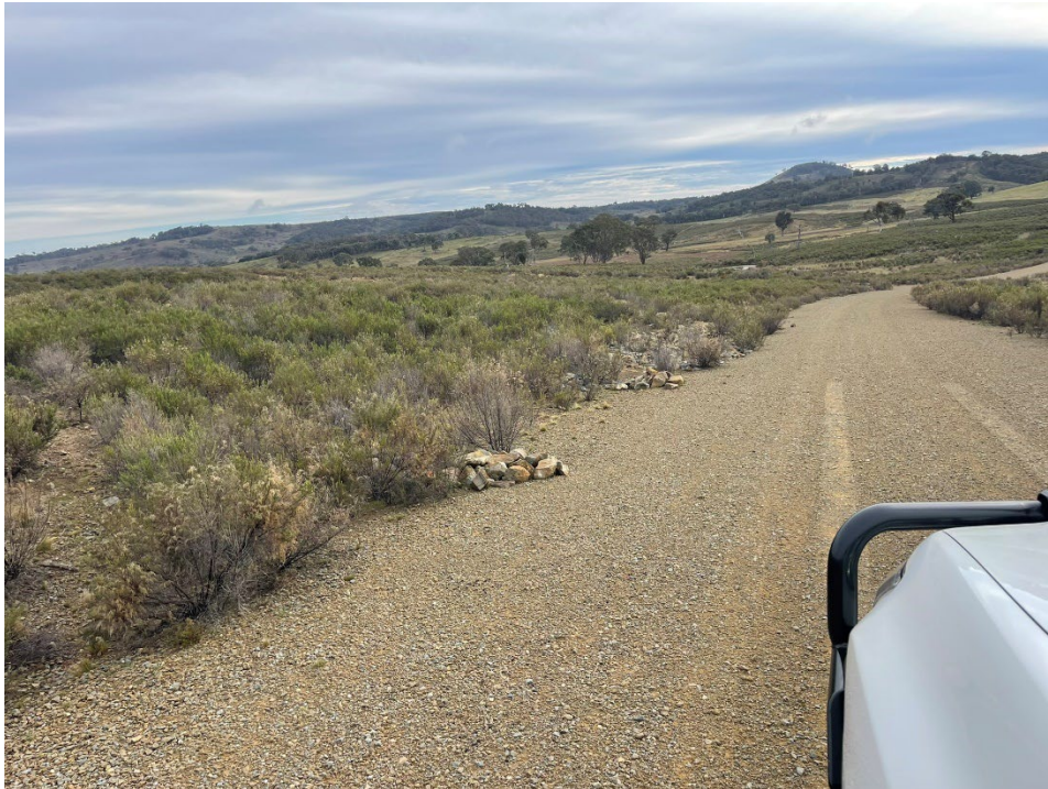
Photo 14 Internal access road showing rock dams to slow surface water velocity.
