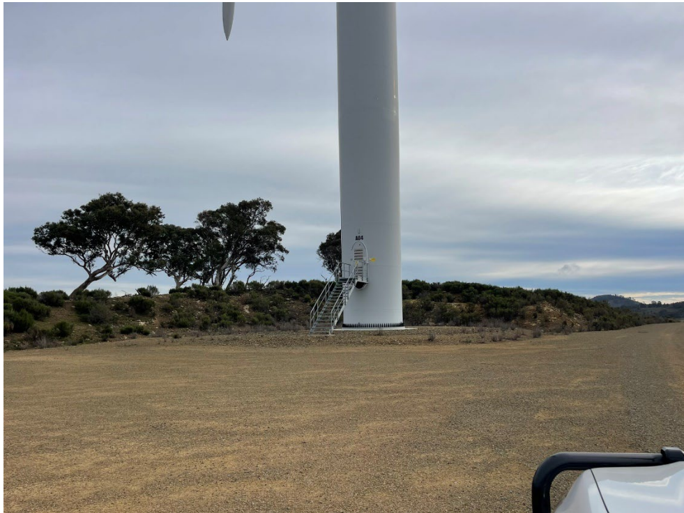
Photo 13 Representative WTG pad showing use of sealed surfaces.
