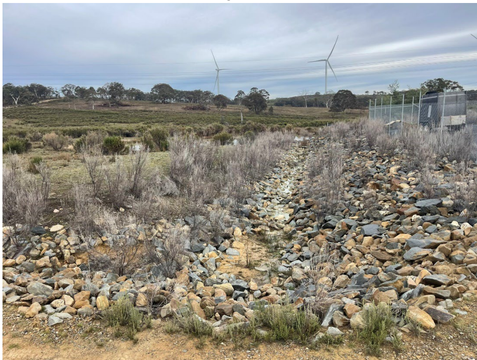
Photo 11 Rock lined swale drains near O&M compound showing weeds that have been sprayed and killed as routine maintenance.
