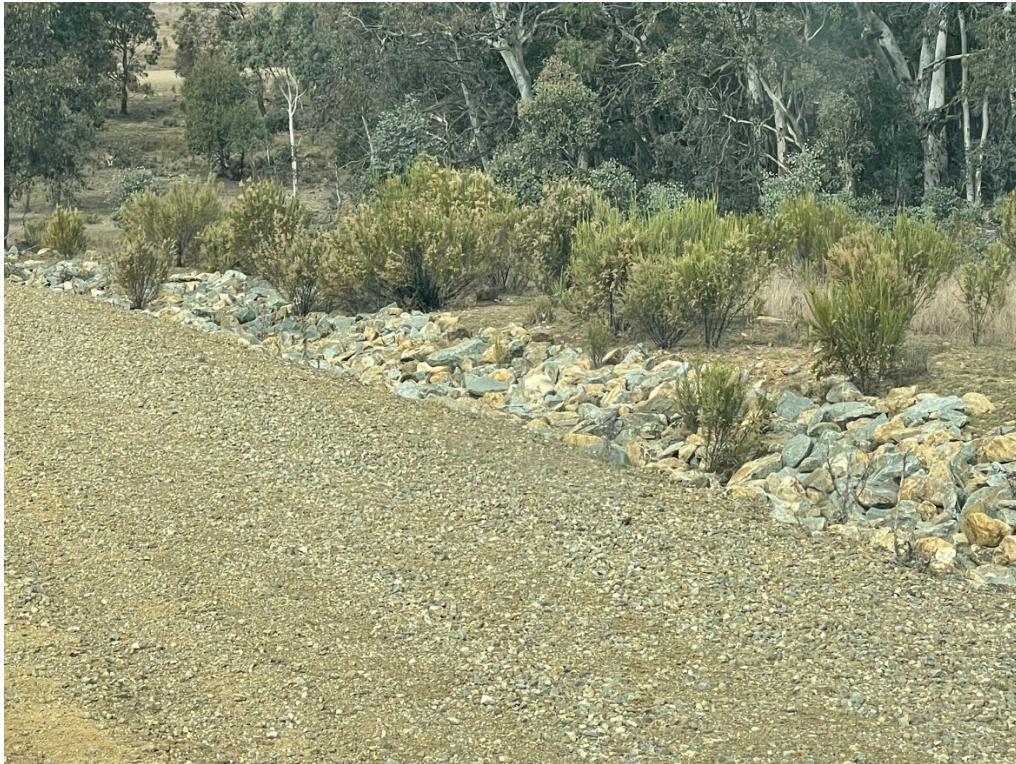
Photo 16 Rock-lined swale drains.
