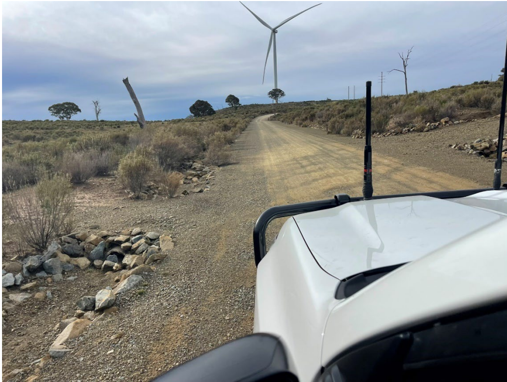
Photo 10 Internal access road showing rock-lined culverts.
