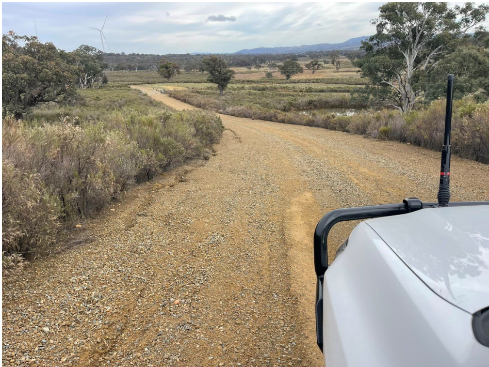
Photo 18 Internal access road showing minor erosion requiring maintenance.
