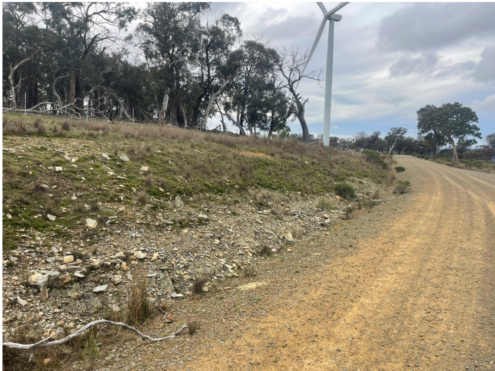
Photo 17 Previously cleared batter showing signs of rehabilitation.
