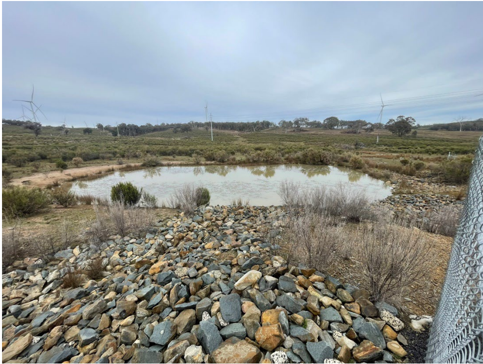
Photo 12 Sediment basin with rip rap used as ERS control.
