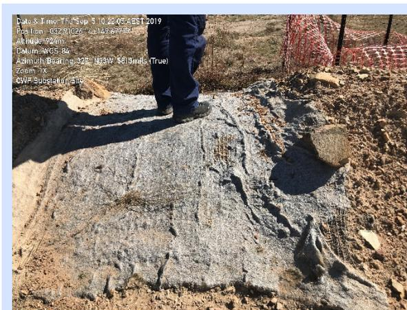
Photo 7. The fabric on the spillway is starting to break down and will erode in a storm event.
