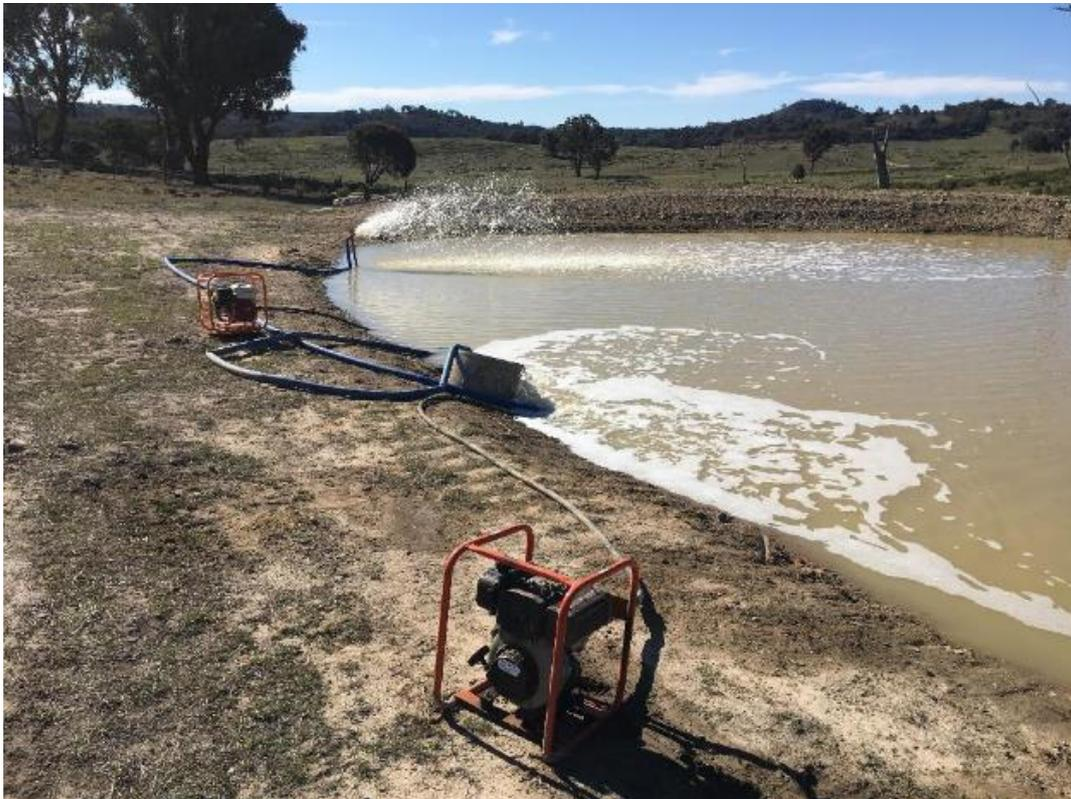
**Figure 8:** Post rain water management (manual floccing in process utilising floc blocks)
