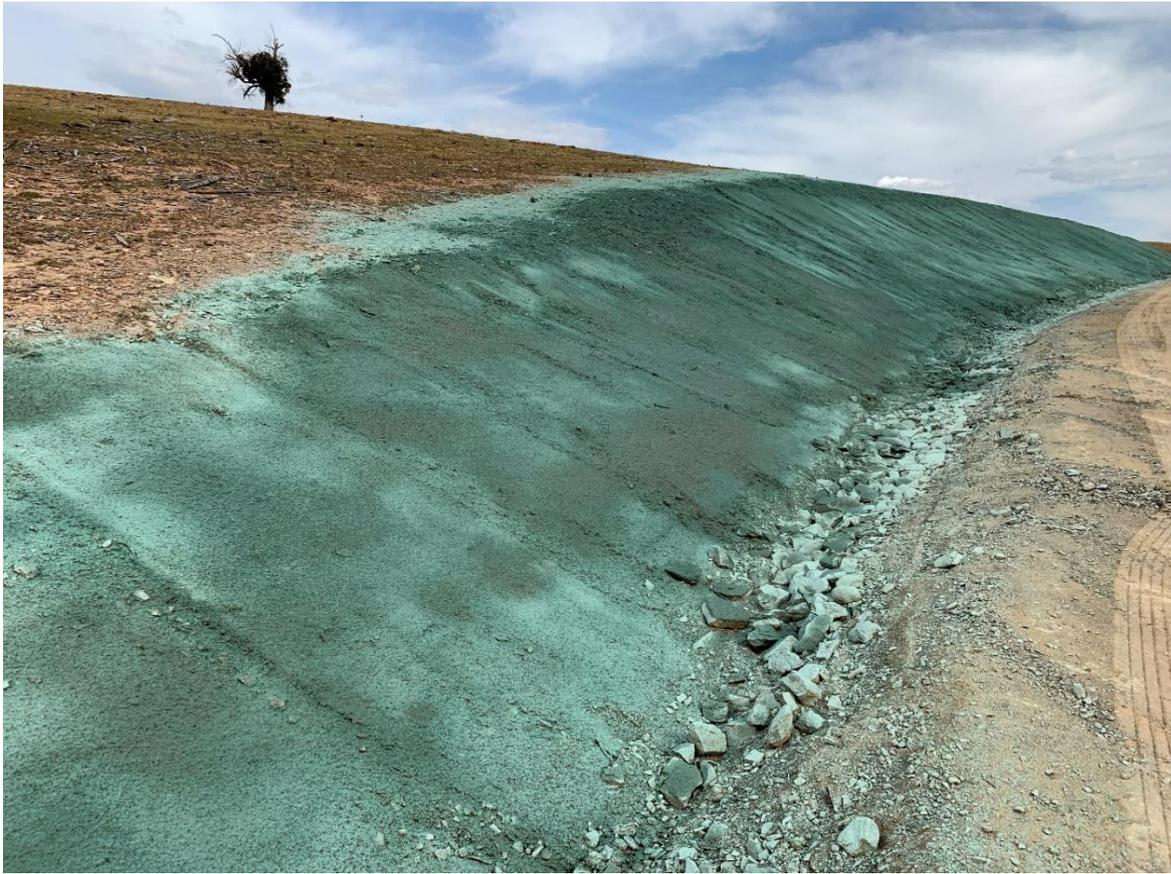
**Figure 1:** Heavy compost blanket applied to batter in CG4 (October 2019)
