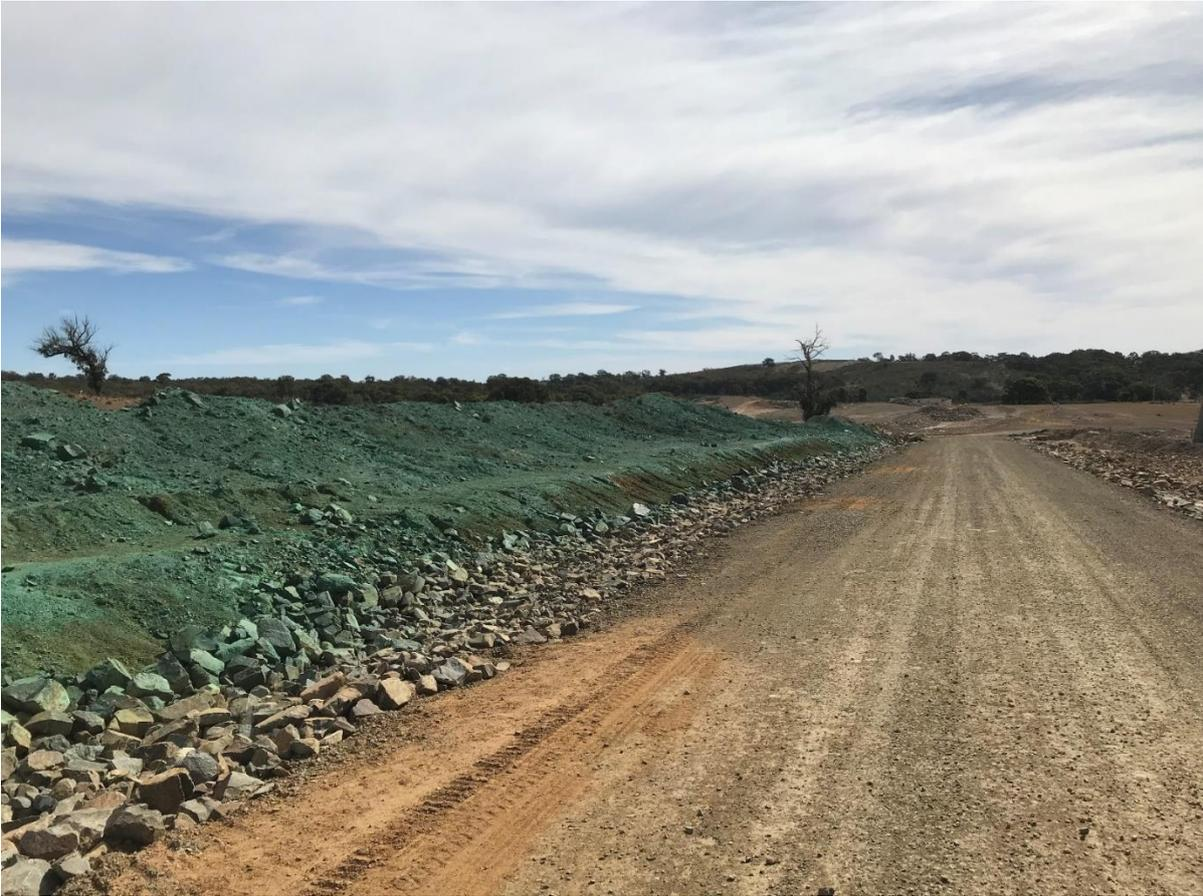
**Figure 7:** Temporary polymer stabilisation (initial coating) applied to Track 5, CG1 higher risk areas where works are currently on hold (March 2019)
