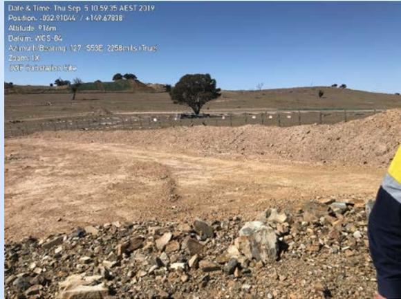
Photo 3. A topsoil bund diverting clean water around the site.
