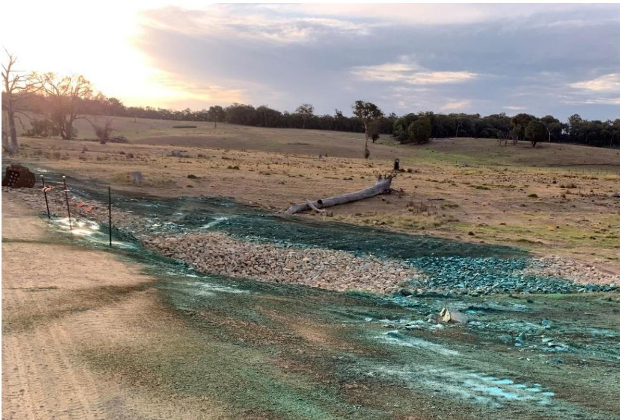
**Figure 4:** Cross drain outlet reset and temporary polymer stabilisation applied in CG4 (October 2019)
