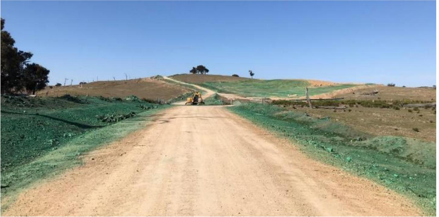
**Figure 5:** Temporary polymer stabilisation (second coating) applied to Track 1, CG1 higher risk areas where works are currently on hold (September 2019)
