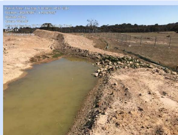
Photo 2. Water Trapped in the sediment trap at the lowest point on site.
