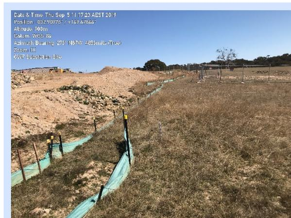
Photo 5. An example where the sediment fence has deteriorated and needs to be replaced.
