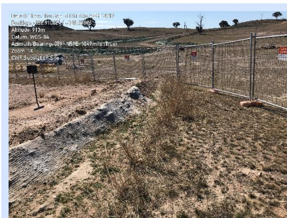
Photo 8. The outlet of the clean water diversion on the south east corner of the site.
