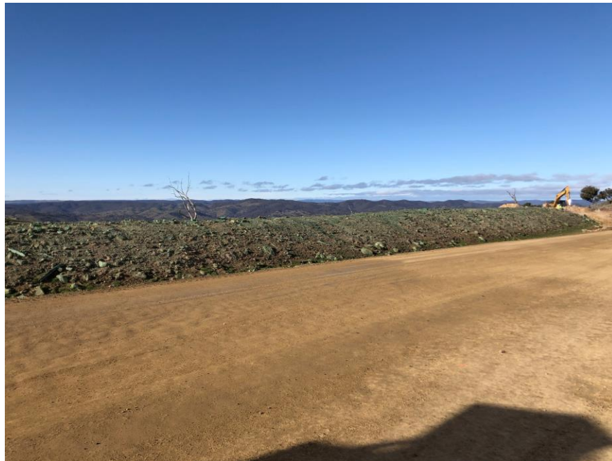
Figure 5 Use of stabilisation polymer onsite
