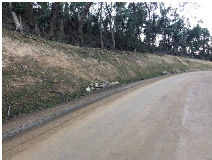
Figure 2 Stabilisation of batter along APR
