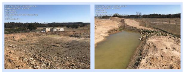
Photo 1. Water trapped in a low point of the excavation near the site offices.
