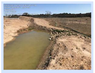
Photo 6. An overview of the sediment trap with rock lined spillway.
