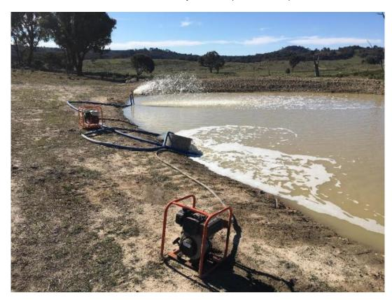
Figure 8: Post rain water management (manual flocking in process utilising floc blocks)
