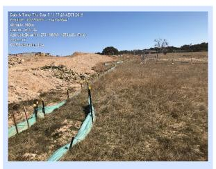
Photo 5. An example where the sediment fence has deteriorated and needs to be replaced.
