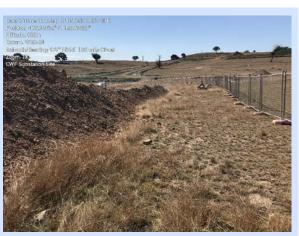
Photo 10. The topsoil bund at the top of the site directing clean water away.
