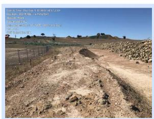
Photo 9. The topsoil bund at the bottom of the site with a flat top that results in concentration of runoff from the surface in rills down the side.
