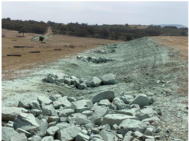
Figure 3: Heavy compost blanket applied to batch plant bench drains (October 2019)
