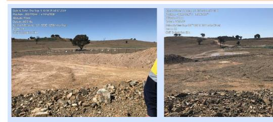
Photo 3. A topsoil bund diverting clean water around the site.
