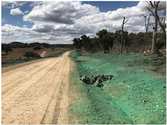
**Figure 6:** Temporary polymer stabilisation (initial coating) applied to Track 1, CG1 higher risk areas where works are currently on hold (March 2019)
