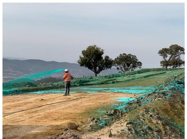
Figure 2: Temporary polymer stabilisation applied to works on hold (Track 6, CG1 October 2019)
