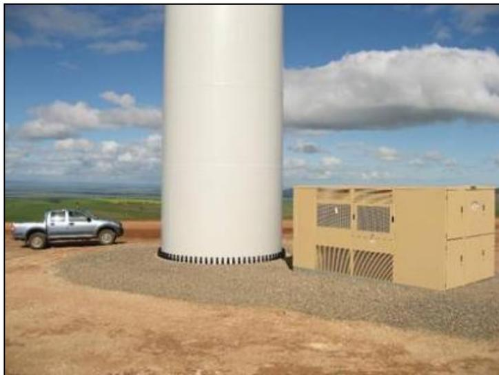
**Image 5: Transformer adjacent to wind turbine**
