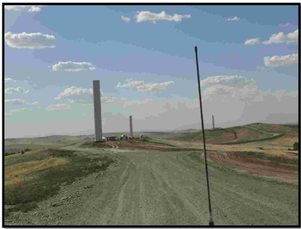
Figure 5.1: Typical unsealed access road within wind farm site
