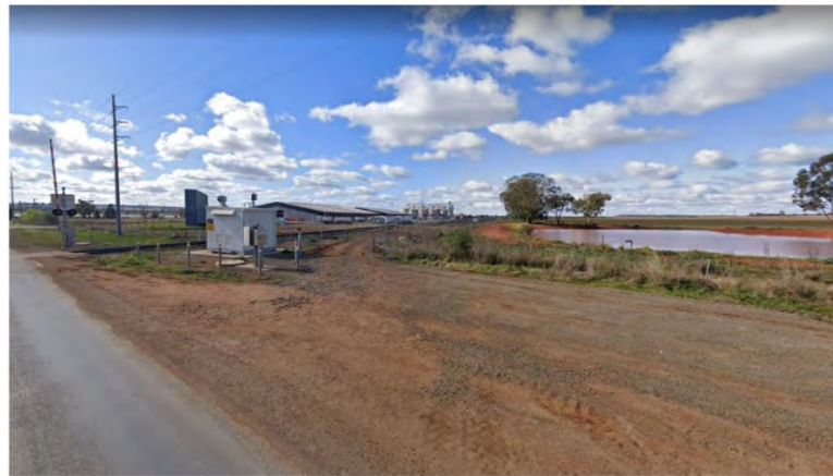
Plate 8: Looking northeast, grain handling facility and inter modal freight terminal
