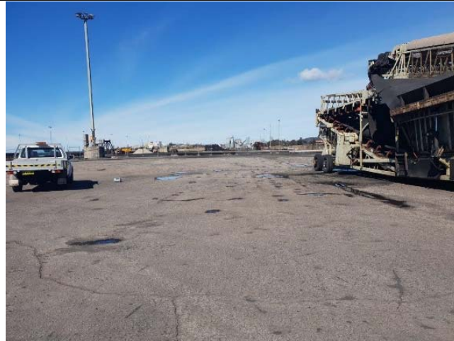
Photograph 3: Looking south towards the paved area of the site, near sample location GBH32 (13/8/2018)
