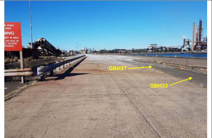
Photograph 4: Looking south at Berth 101 and proposed excavation area. GHD borehole locations GBH33 and GBH37 were drilled in the area shown (13/8/2018)
