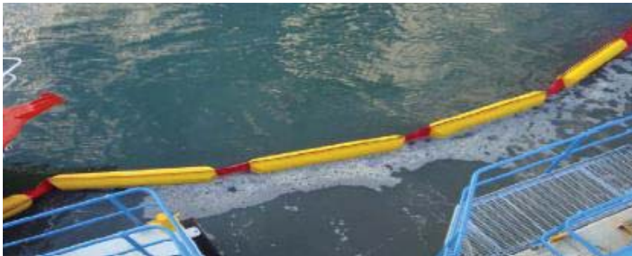
Figure 5 Example of a silt curtain surrounding a dredging operation
