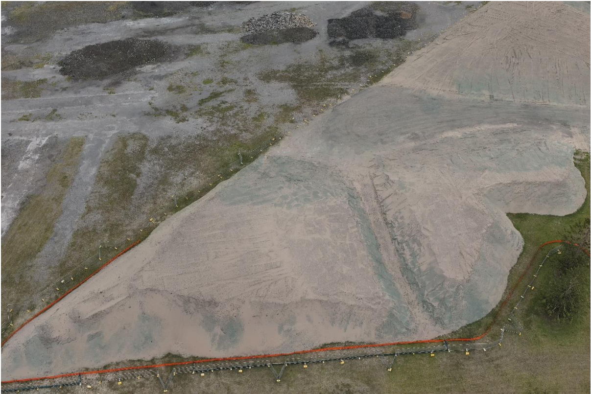
Photograph 1: View of Outer Harbour stockpiles showing polymer application and sediment controls in place.
