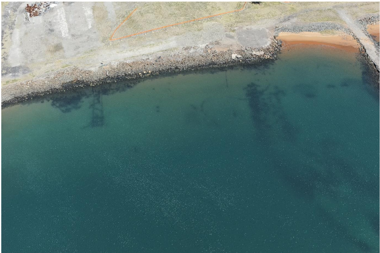
Photograph 2. View of sediment fence installed at the Outer Harbour site, facing west. Captured 22/09/2021
