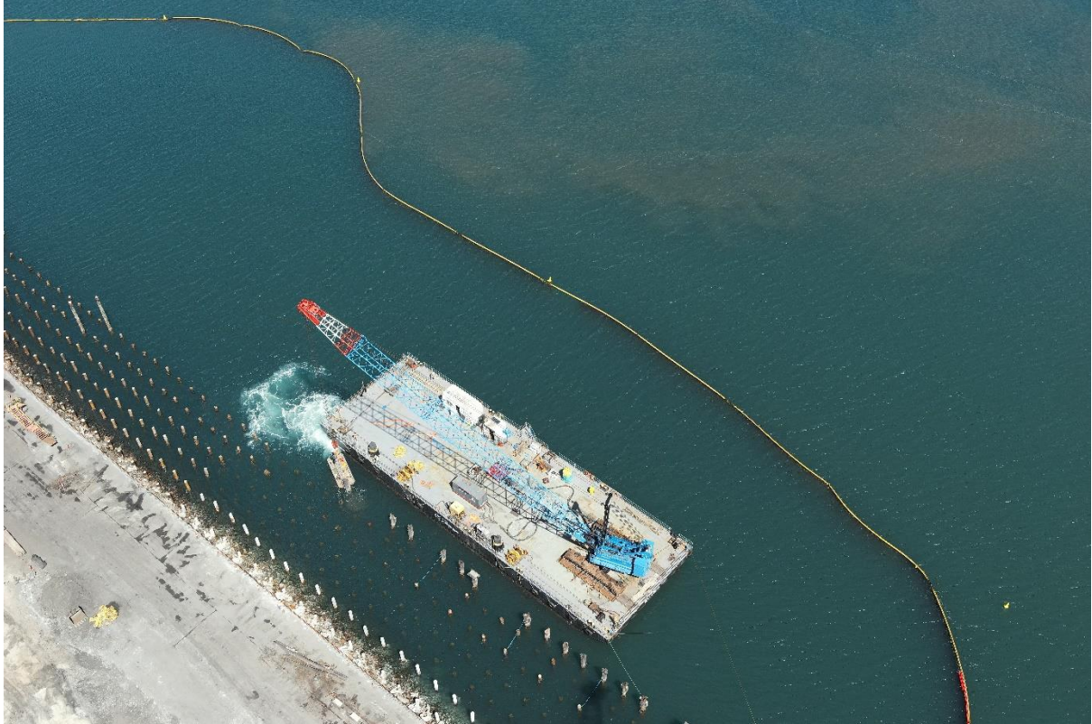
Photograph 1. View of pile removal barge and silt curtain at Berth 101. Visible sediment as a result of a recent ship movement. Facing west. Captured 22/09/2021.
