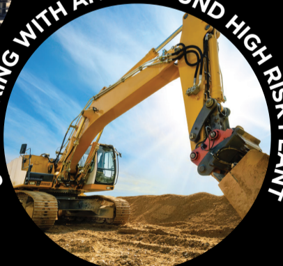
5. EXCAVATIONS AND TRENCHES
