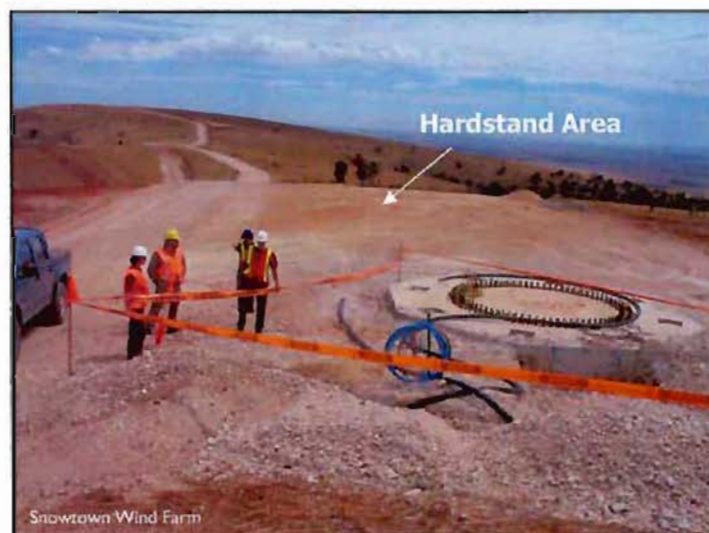
Image 3: Typical Hardstand area adjacent to a Rock Anchor footing
