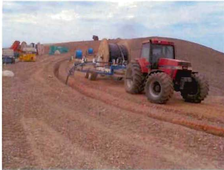
Image 7: Laying underground electrical cable within road network
