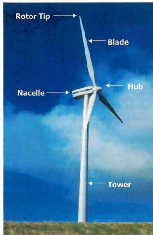
Image 1: Component Parts of a Wind Turbine
