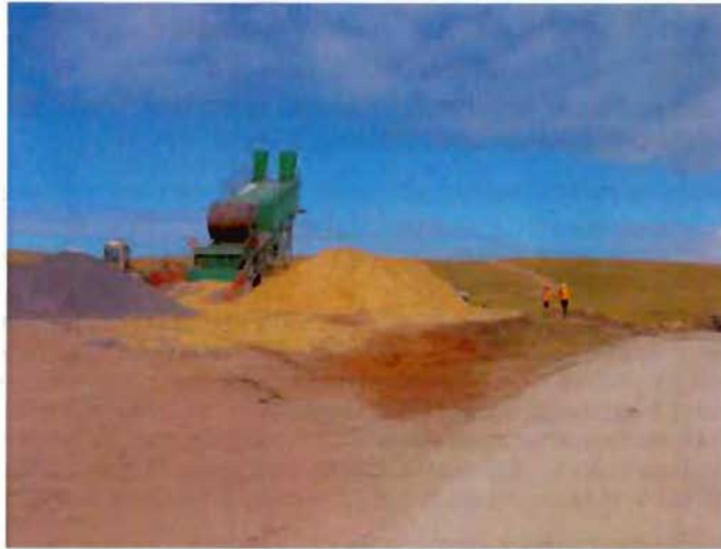
Image 9: Temporary on-site concrete batching plant
