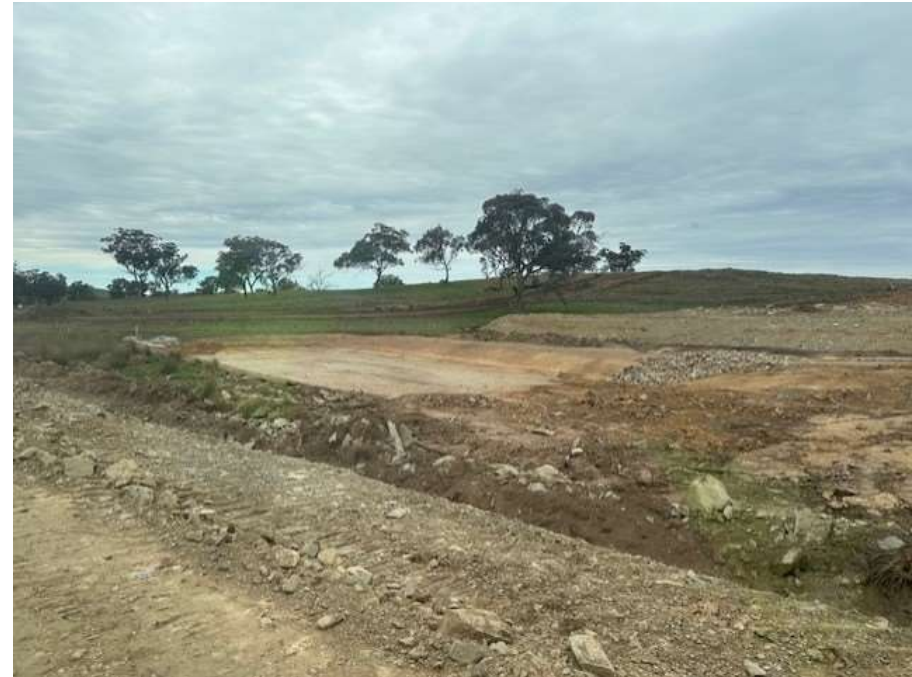
Civil Area 03 – GE Pad Sediment Basin
