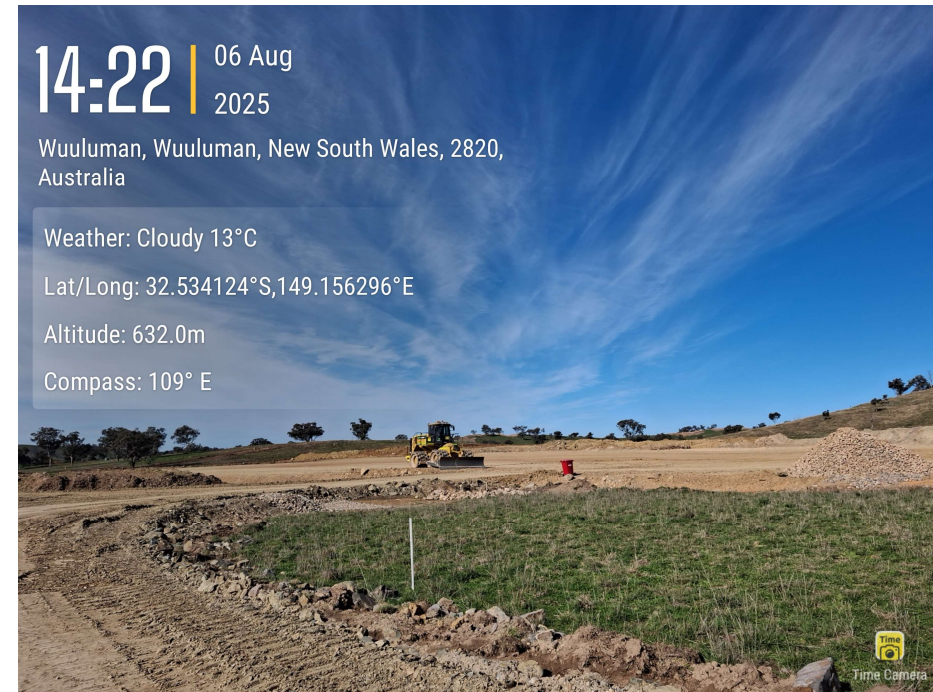
Civil Area 03 – GE Pad Cut Fill
