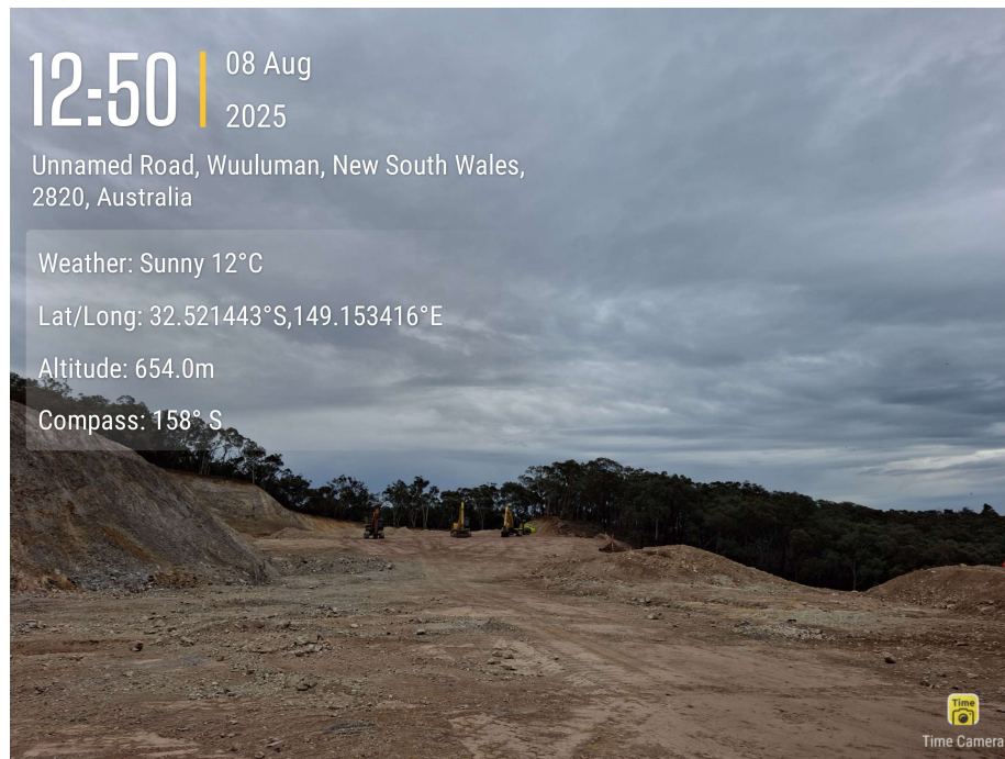
Civil Area 03 – WTG-26 Cut Fill
