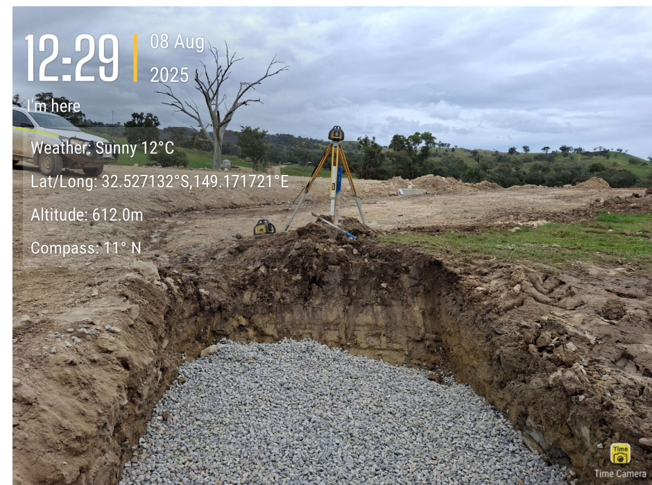
Civil Area 05 – SW-5-1-2 Laser
