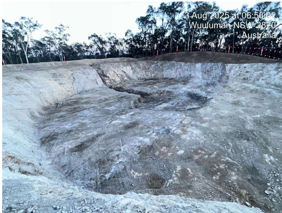
Civil Area 01 – WTG-09 Foundation
