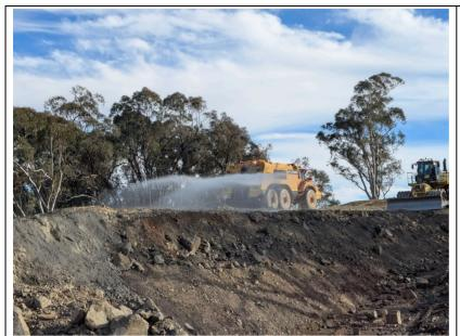
Pad nine (9), civil works ongoing. Dust suppression was observed to be undertaken using water carts at the time of inspection. No visible dust from ongoing earthworks at the time of the inspection.
