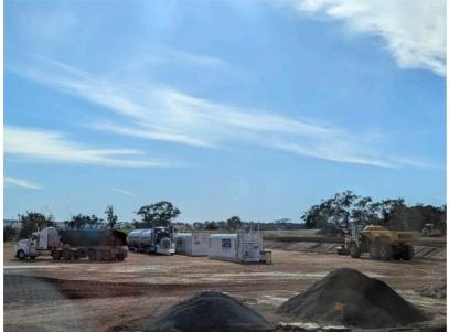
Workshop and site laydown area establishment in progress. Two (2) 70,000L fuel tanks, self-bunded were delivered (relocated). Appropriate spill containment equipment and firefighting equipment was also sighted to be in place in the laydown area.
