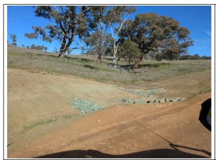
Clean water diversions and rock check dams in place in accordance with approved erosion and sediment control plans endorsed by the CPESC.
