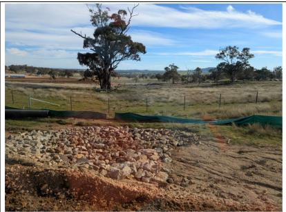
Boundary fencing was observed to be in place with erosion and sediment controls including rock checks and sediment fences.
