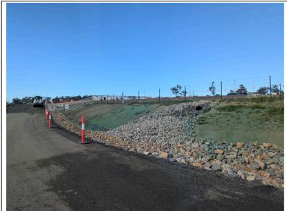
Evidence of polymer or soil binder application and rock placement for erosion and sediment control was observed.
