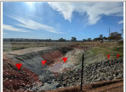
Erosion and sediment controls were observed to be in place around access tracks and swales in accordance with the approved erosion and sediment control plans.
