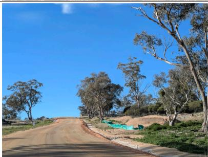
Topsoil stockpiles were observed located within the approved project boundary and appropriate sediment controls were in place around the stockpiles.
