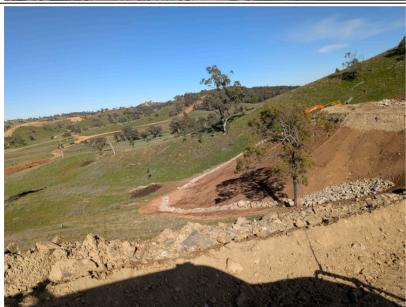
Facing west, photograph showing embankment being covered with topsoil and rock protection in place downslopes for sediment control. All works were contained within the approved project boundaries as per visual observations.
