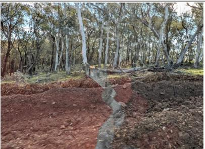
Mulch berms were observed to be installed around the work areas. Sediment controls were observed to be in place.
