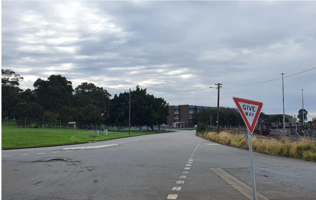
Figure 6 – Selwyn Street, looking North towards Port of Newcastle
