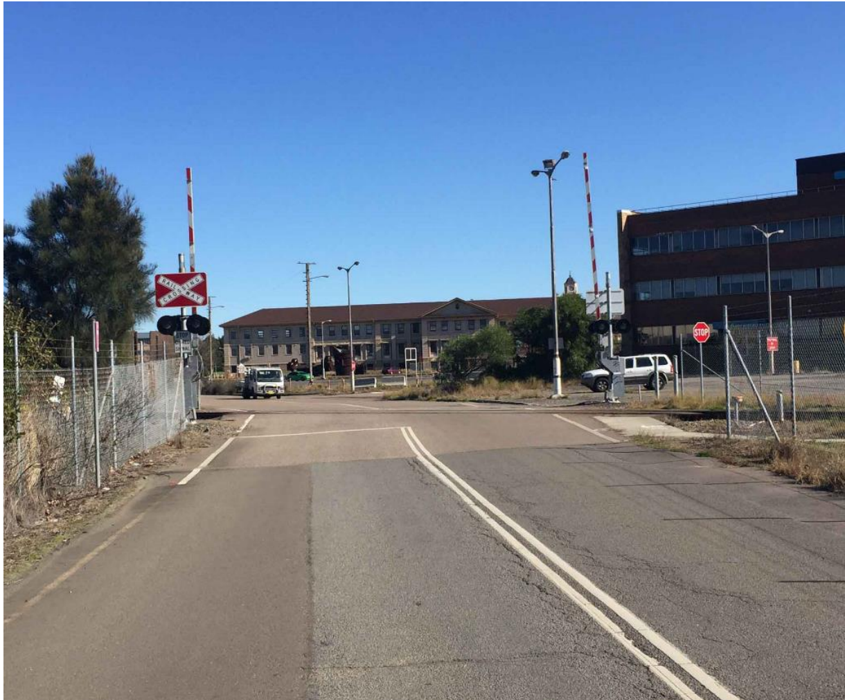
Figure 12 - Rail crossing over Selwyn Street
