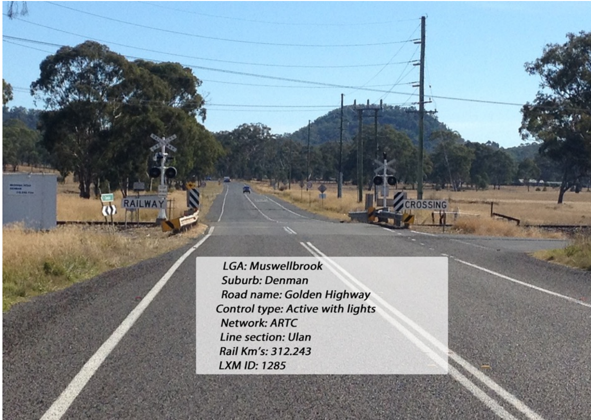
Figure 29 - Denman Rail Crossing
