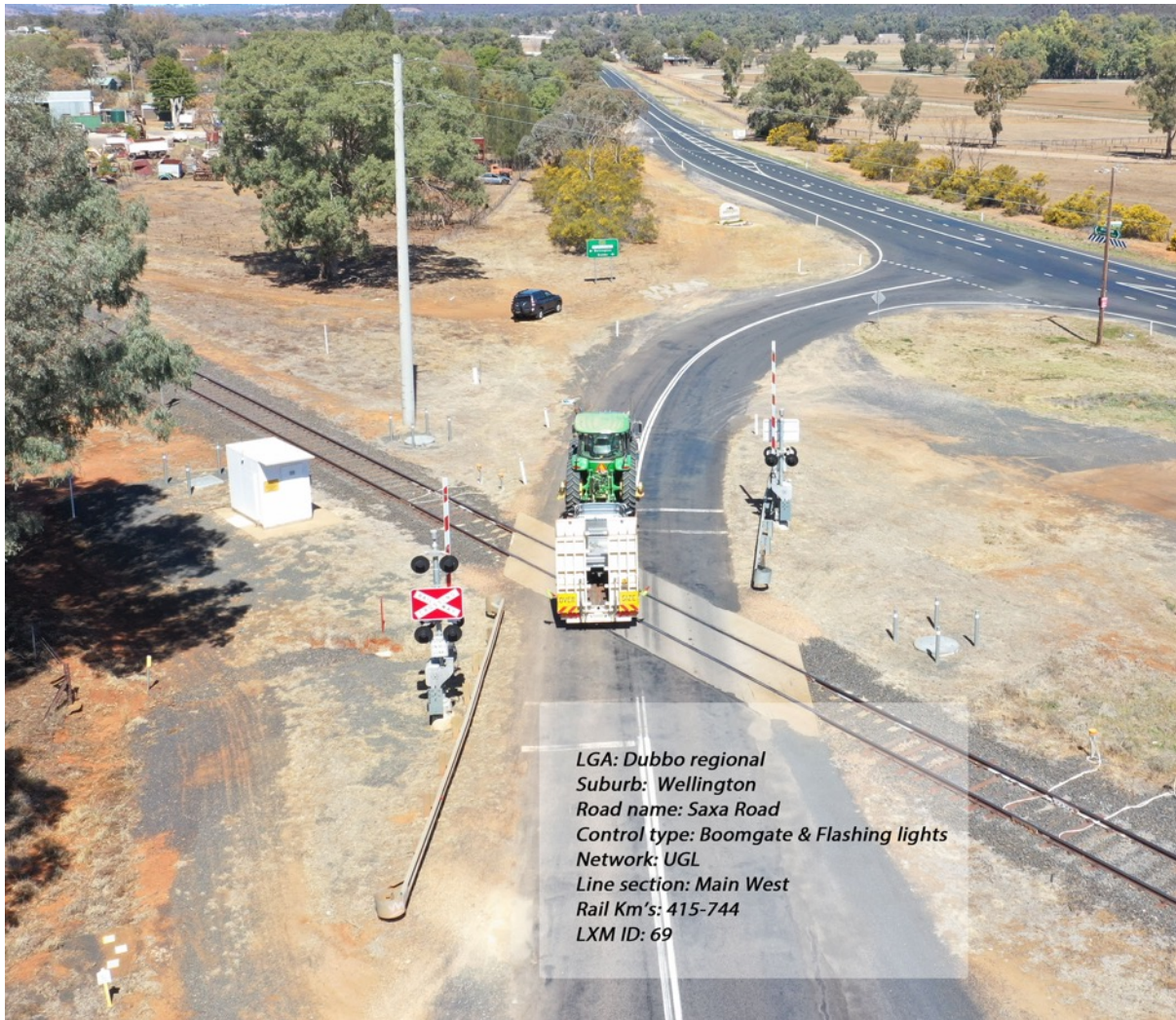
Figure 35 - Saxa Road Rail crossing at Wellington
