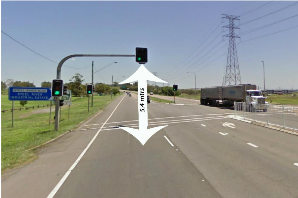
Figure 14 - Standard Overhanging Traffic Signals
