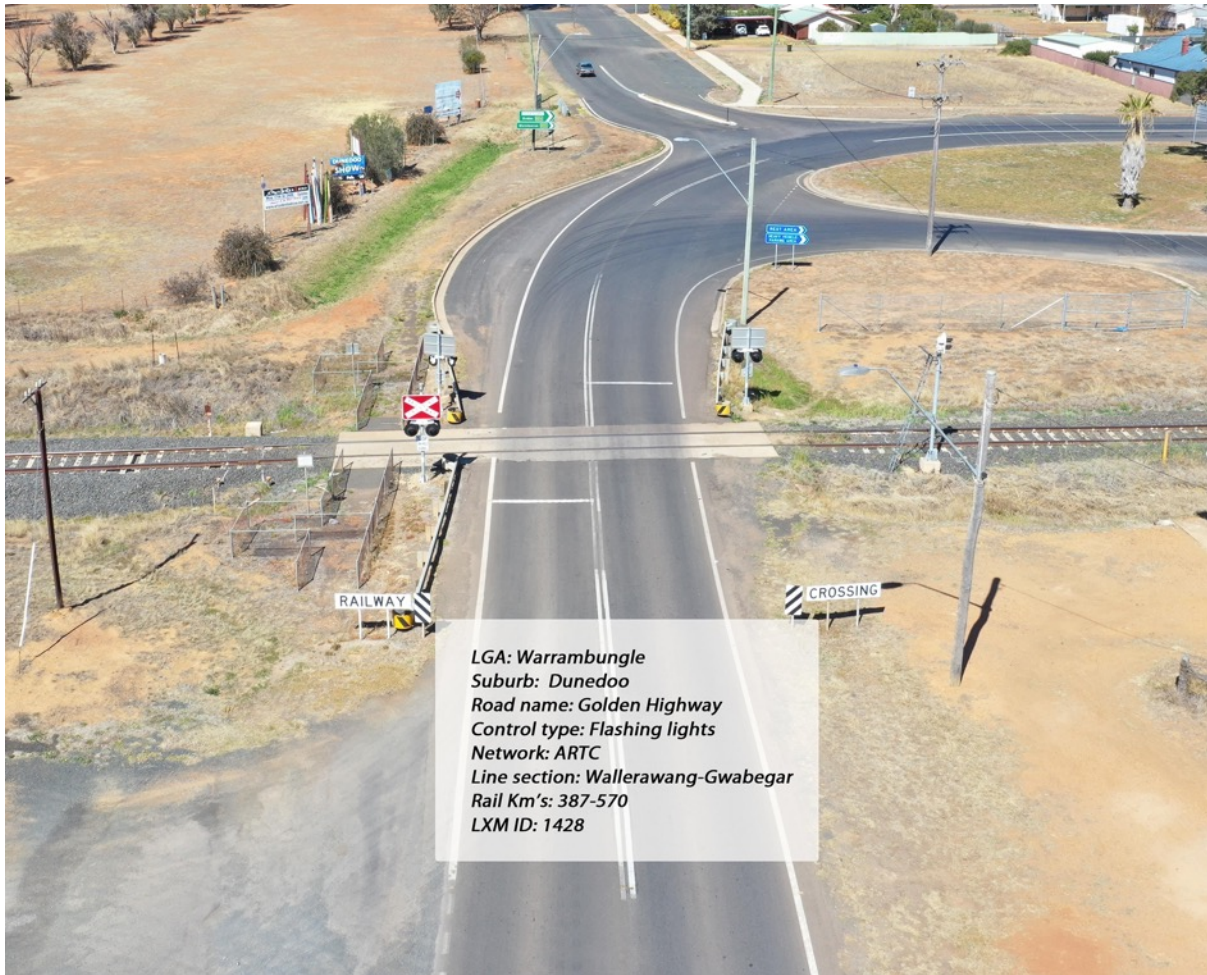
Figure 32 - Golden Highway rail crossing at Dunedoo
