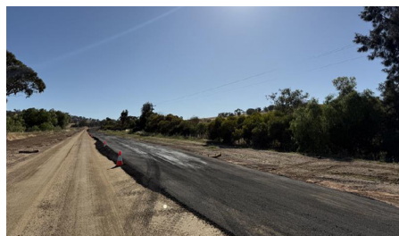
Images: Installing a layer of road base on Twelve Mile Road
